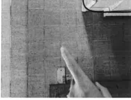
15- VERTICAL CRACK
