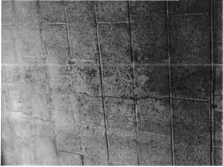
8- VERTICAL CRACKS @ 4' O.C. TYP.
